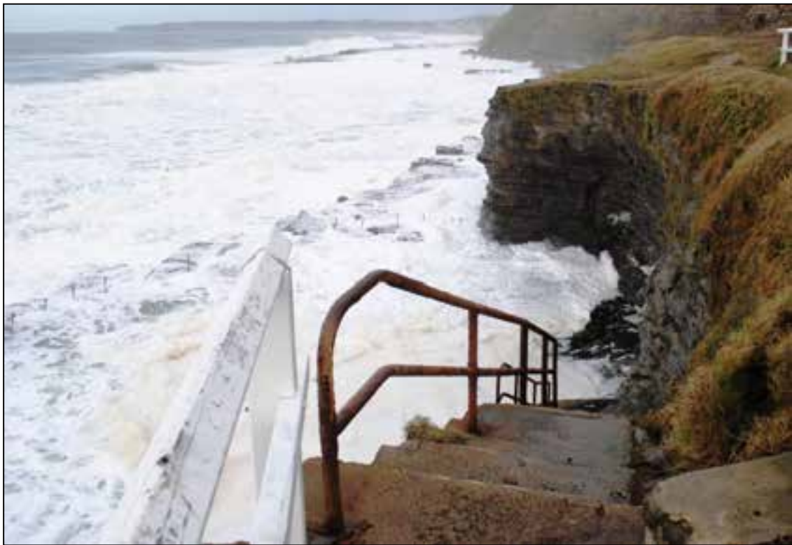
Figure 4 Bogie Hole inundated by wave action, with loss of amenity approximately 1¼ hours past a 1.3m high tide; approximating BMT WBM modelled year 2100 mean sea level.
