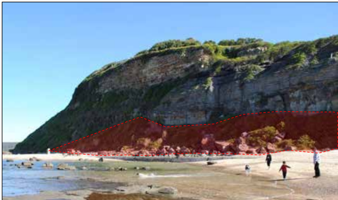
Figure 19 Geo-hazard #18 – Lloyd Street cliff face instability resulting in rock falls and mixed debris slide debris, shown in red. Hazard affects beach and southern end of Merewether Baths.
