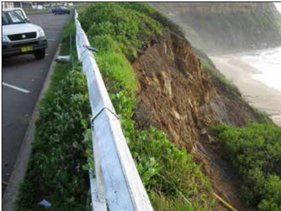
Figure 17 Geo-hazard #16b – Accelerated weathering/regression of the Dudley Seam & low strength rocks exposed mid-slope of cliff/slope are resulting in upper slope landslides threatening Bar Beach Car Park along crest of cliff/slope.
