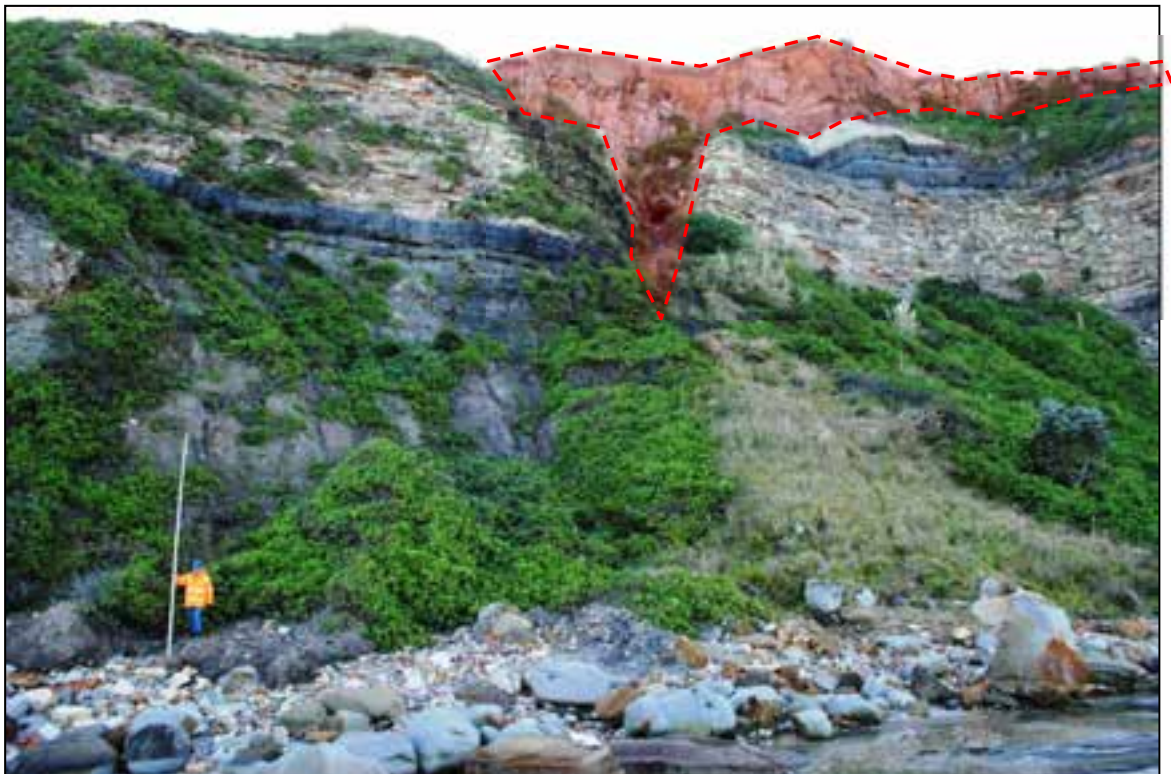
Figure 20 Geo-hazard #19 – Accelerated cliff face retreat along Fault line & cliff top, shown in red. Edge of cliff crest comes within 3-6m of existing cliff top residences.
