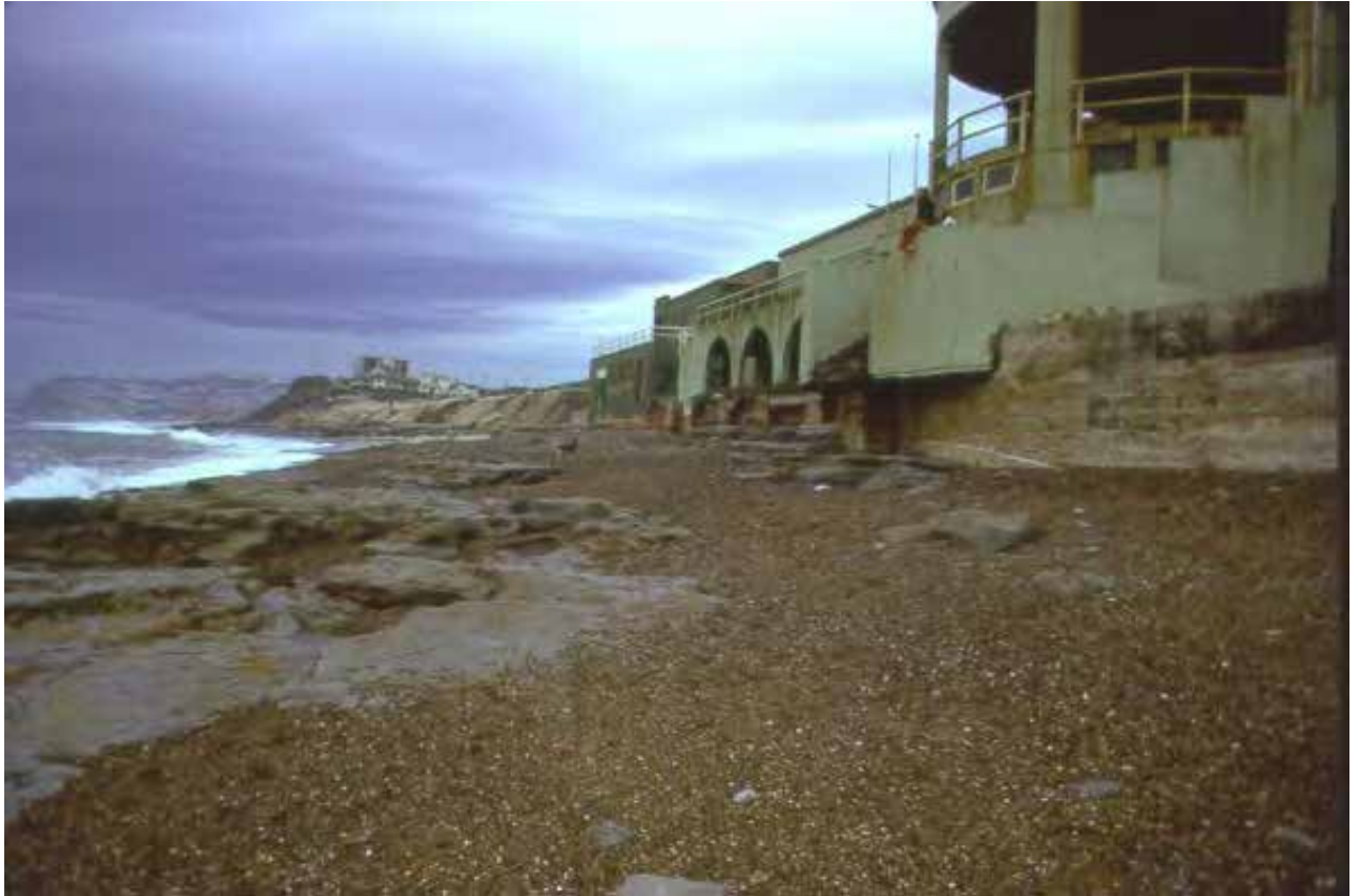
Figure 4-3 Bar Beach (centre) Erosion Extents Following Severe Storms circa 1974
