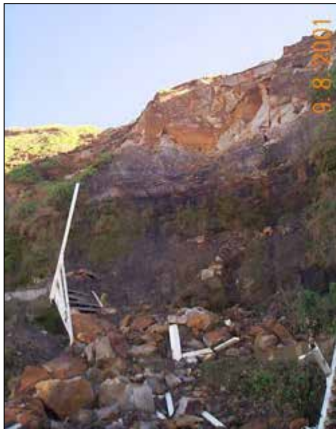
August 2001 wooden stairs to SGB destroyed by a rock slide.
