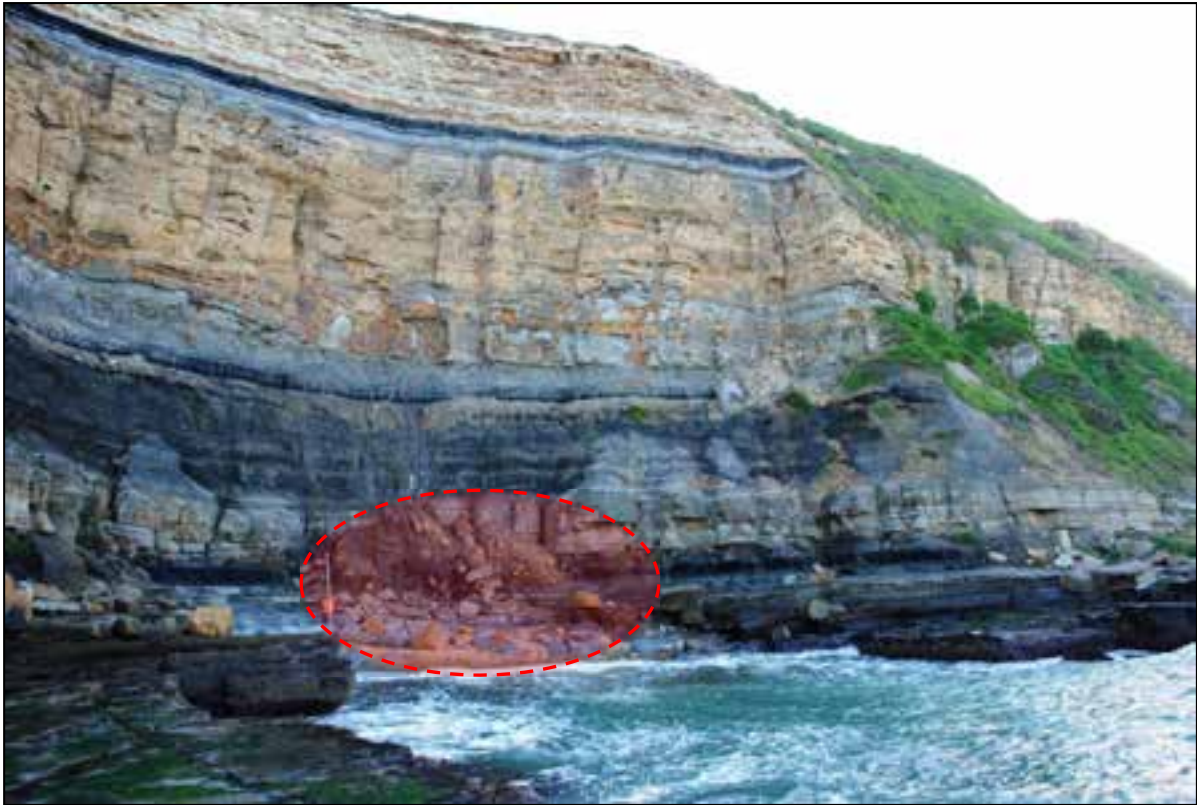
Geo-hazard #14 – recent rock fall(s) and debris slide circled, covering narrow rock platform at toe of cliff face.
