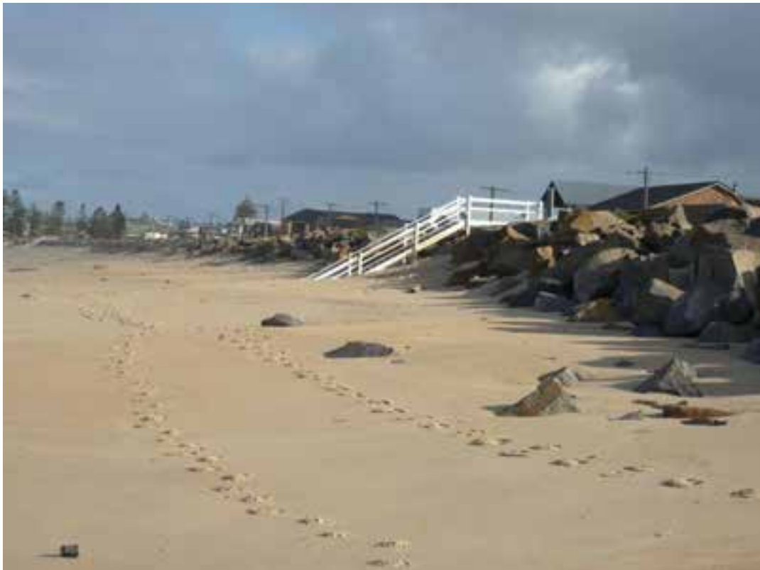
Figure 4-20 Stockton Beach (June 2011) With Sand Accreted Onto Mitchell St Seawall
