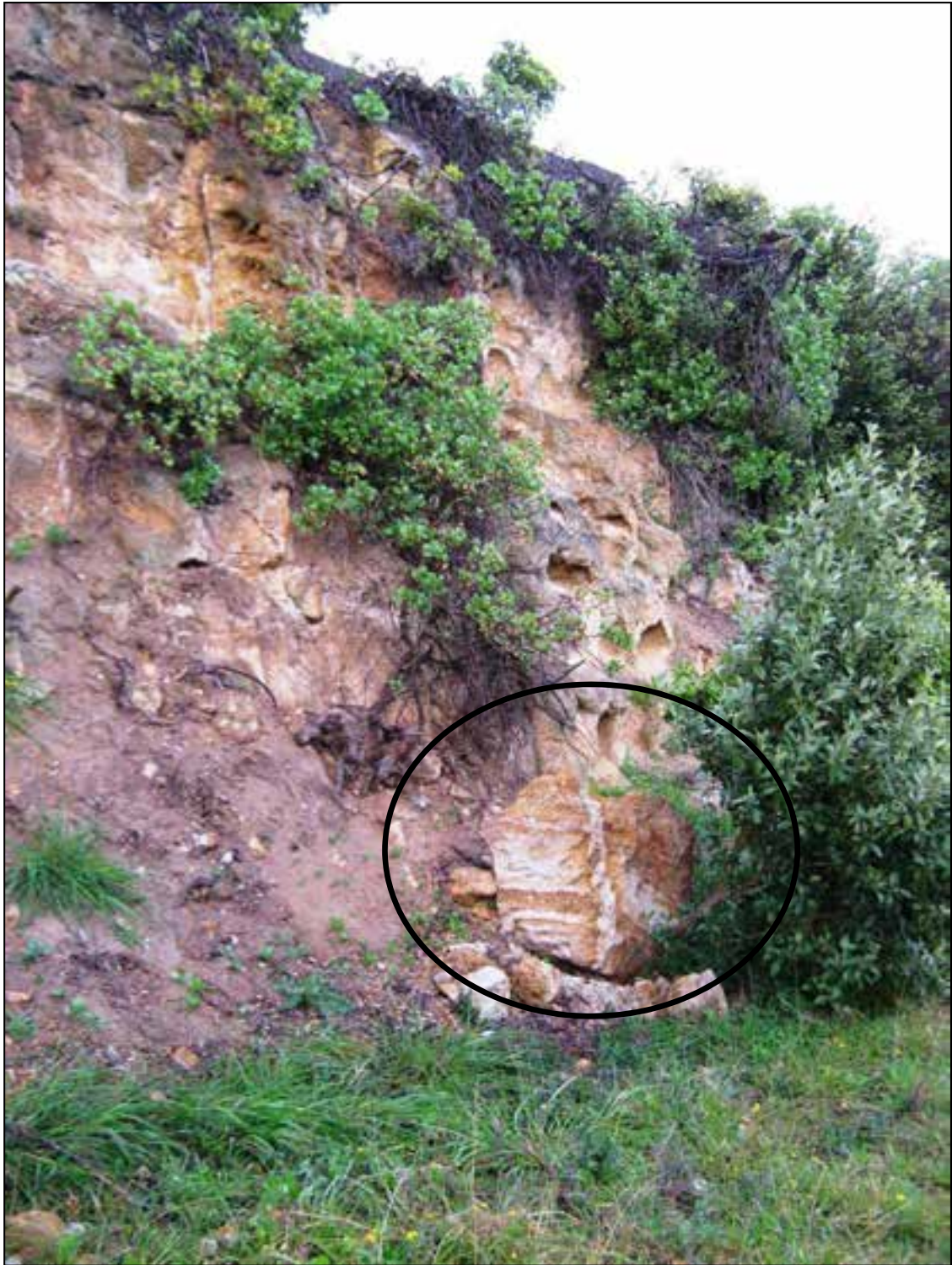
Figure 22 Geo-hazard #21 – Rock falls from north face of Obelisk Hill. Fallen block ~1m in dimension circled. Observed rock falls have come to rest within 2m of rock face.
