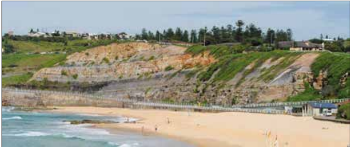
Figure 9 Geo-hazard #8– Rock falls from South Newcastle Cliff face.
