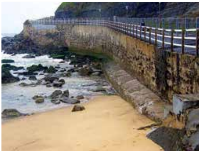
Plate 2.10. South Newcastle beach, old vertical rendered stone revetment protects the now closed section of Shortland Esplanade immediately behind the beach. Photo: Coastal Environment 30/04/2011.
