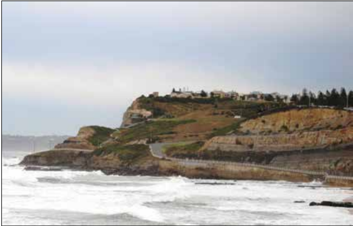
Figure 3 Bogie Hole & South Newcastle sea wall subject to constant wave action; approximately 1¼ hours past a 1.3m high tide, approximating BMT WBM modelled year 2100 mean sea level.
