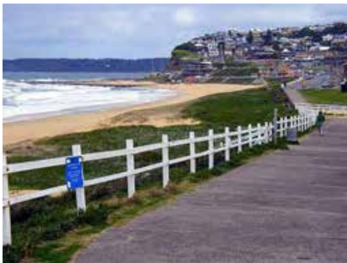
Plate 2.5. A sloping rock armoured revetment extends from the boat ramp at Merewether SLSC to the northern extent of the Dixon Park SLSC. This wall, constructed in the 1970s is buried beneath the existing dune. Photo: Coastal Environment 30/04/2011
