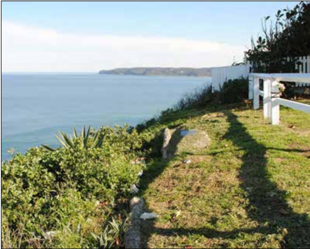
Geo-hazard #18 – Lloyd Street cliff / slope erosion along crest is within 2-3m of the boundaries of cliff top development
