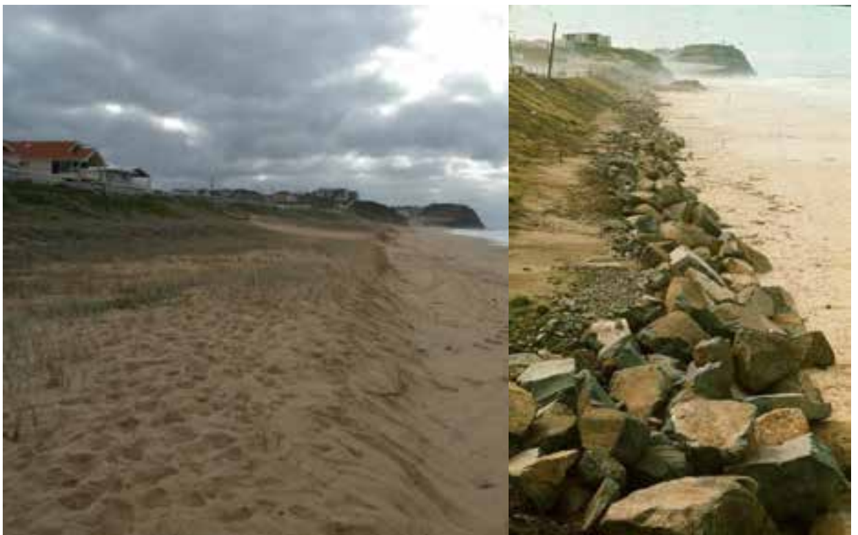
Figure 4-2 Merewether to Dixon Park (2011) – Well developed dunes now overlay seawall (right)
