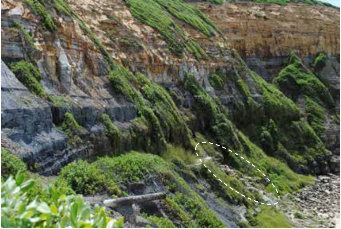
Figure 8 Site of destroyed wooden steps (circled) above Susan Gilmore Beach in 2012
