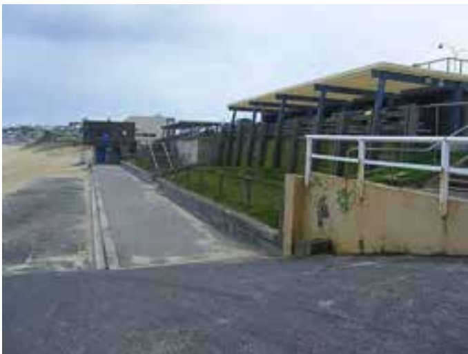
Plate 2.8. View north along the Bar Beach foreshore. The low level promenade is at the left. The lifeguard tower is in the background and the Cooks Hill Surf Club beyond. Photo: Coastal Environment 30/04/2011.
