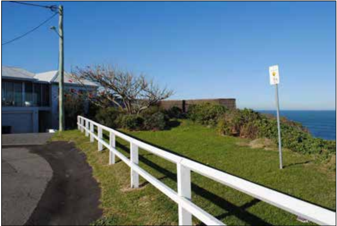
View of cliff top development above Geo-hazard # 19. Right hand-side panel of Brushwood fence in centre of picture is 'suspended' over ragged bare rocky cliff edge.
