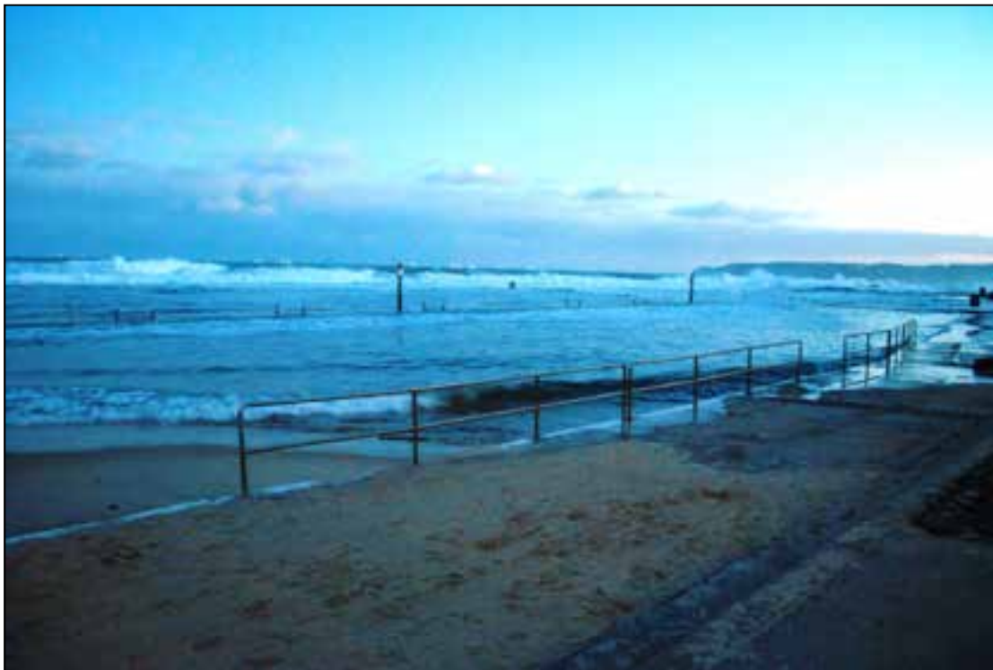
Figure 6 Merewether Baths inundated with loss of amenity, approximately 2 hours before a 1.9m high tide. Illustrates BMT WBM modelled year 2100 mean sea level.
