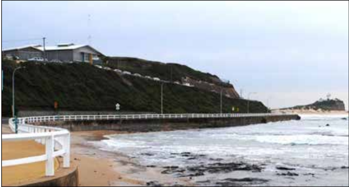
Figure 1 Fort Scratchley's Eastern Sea Wall will be exposed to increased wave action, as shown 1½ hours past a 1.3m high tide, approximating BMT WBM modelled year 2100 mean sea level.
